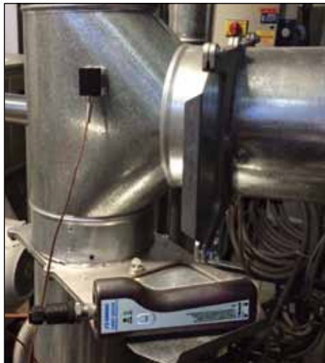
Figure 5: 88401K magnetic probe mounted to a vacuum exhaust system
