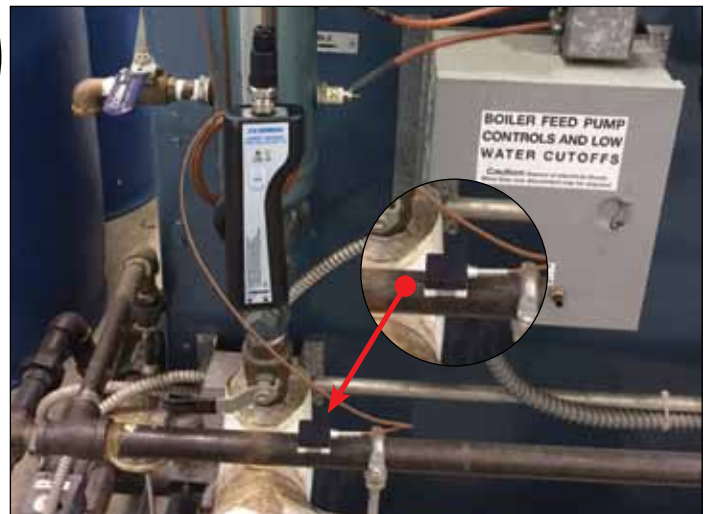
Figure 8: 88401K probe measuring pipe temperature
